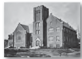
10 2730 EAST 31ST STREET: HOLY TRINITY LUTHERAN CHURCH
