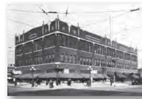
8 2700 EAST LAKE: COLISEUM BUILDING/ FREEMAN'S DEPARTMENT STORE
